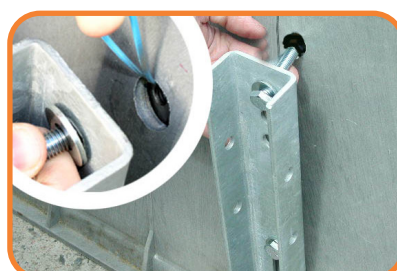
Fit bracket over bottom screw. Insert top toggle and fix bracket with screw and washer
