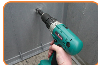
Drill 22mm holes with holesaw or flatbit
