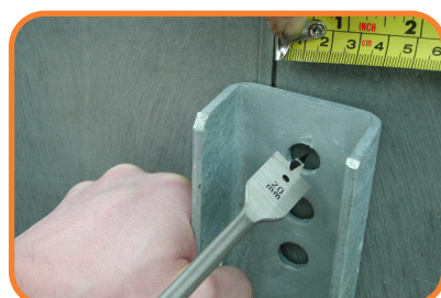
Use step as a template to mark 2 holes 15mm from edge of rib
