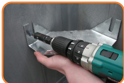
Use step as a template to mark 2 holes
