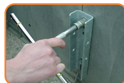
Tighten both screws
