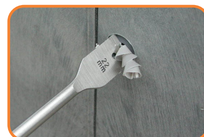
Drill 22mm holes with holesaw or flatbit
